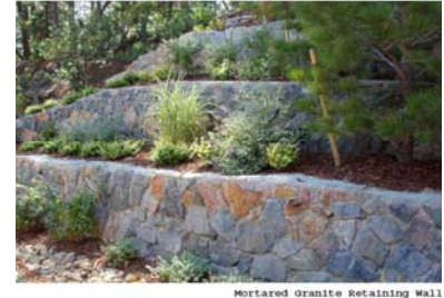
Mortared Granite Retaining Wall
